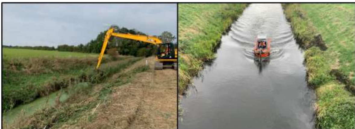
Photos 3/4: Weed control on Carr Dyke between Timberland and Martin using an excavator and weed basket (left); weed control on the South Forty Foot using Conver weed boats (right)
